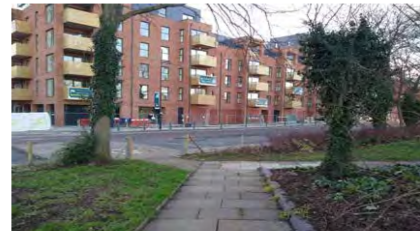
Recently completed Riverside Baths
