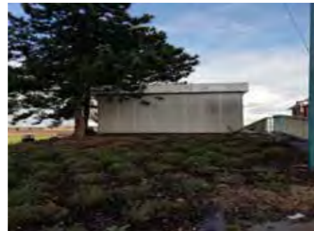
4. Embankment to south-east boundary
