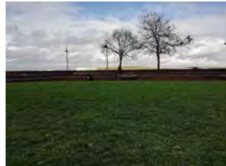
6. View north-east and flood defence wall
