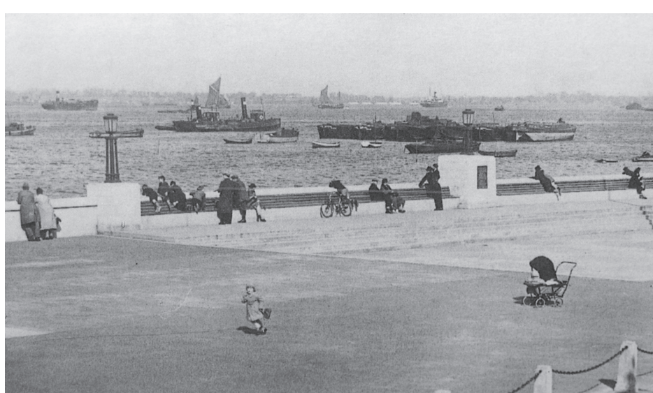
Following the demolition of the Gaze and Cannon Flour Mill, Erith Riverside Gardens were opened to the public in the early 1940's
